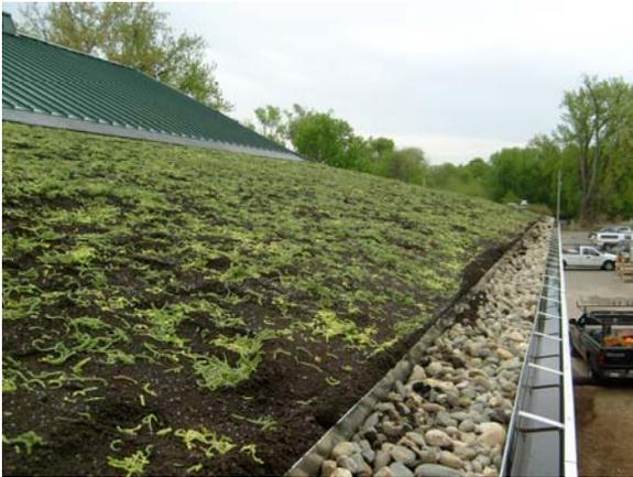
This green roof project involves a 13,000 square-foot area with a 25 percent slope. Design includes sturdier roof framing, a thick waterproof membrane to protect the roof, and four inches of bio-engineered growth media that is planted with eight varieties of Sedum to reduce stormwater runoff from the roof. In addition to capturing rainfall, the roof improves energy efficiency within the building, lowering heating and cooling costs.
